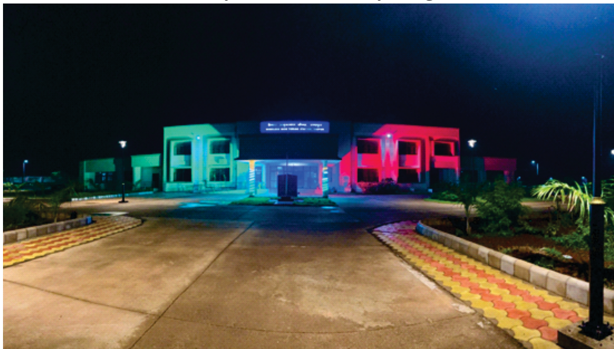
Newly constructed office building of WMS Raipur
